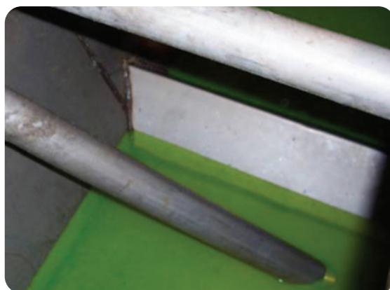
After using QUINTOLUBRIC®, the tank has been clear and bacteria-free for 5 years and has never been cleaned.
